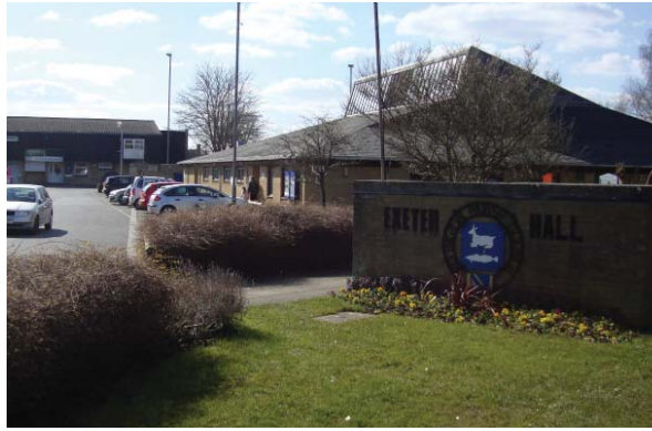
Figure 2.4 Village Centre - Exeter Close
