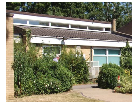
Figure 2.16 Health centre, Exeter Close
